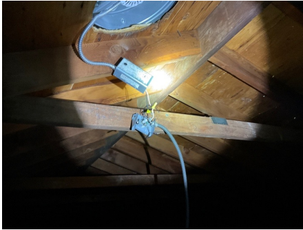
Electrical Splices
